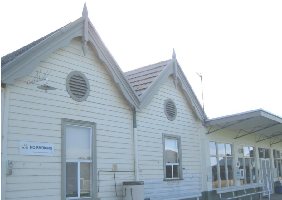
Beachport Railway Station, in 2018, now the Beachport Bowling Club rooms. Tom Clark would have known this station, & the workshops where his father worked.
