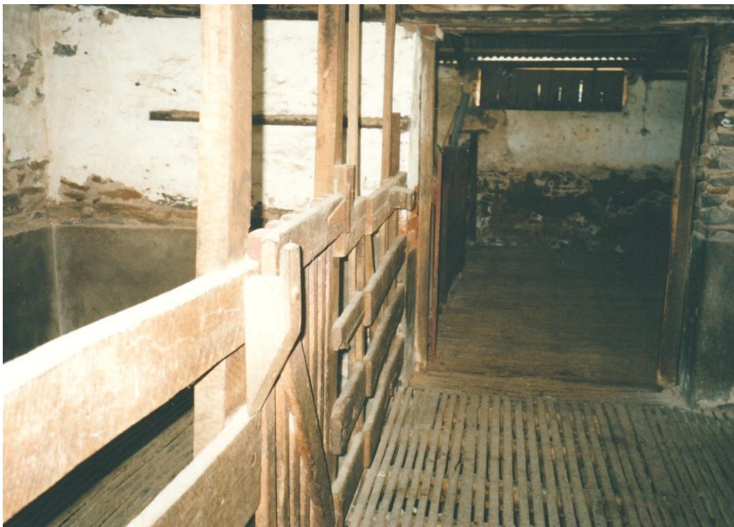
Showing lath floor of shearing shed
