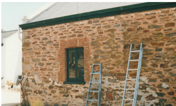
Original stonework on single-men's quarters, Highland Valley station (Photo: W.Baker 2002)
