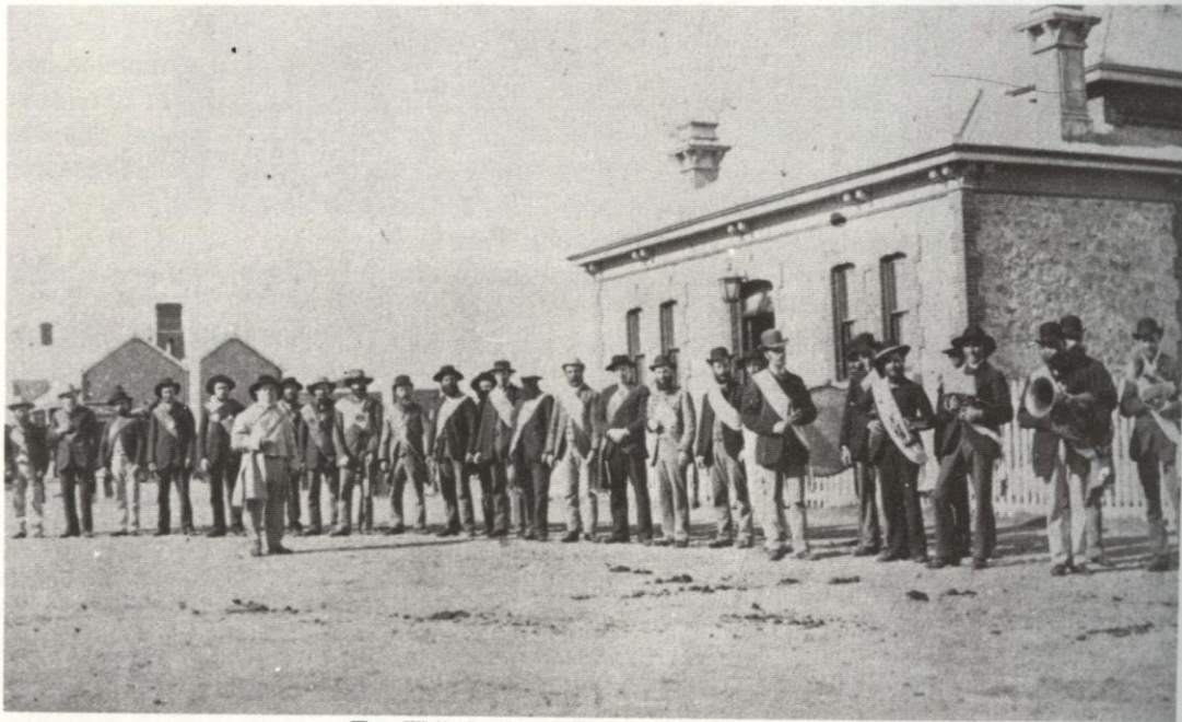
Two Wells Institute after the erection of the fence
